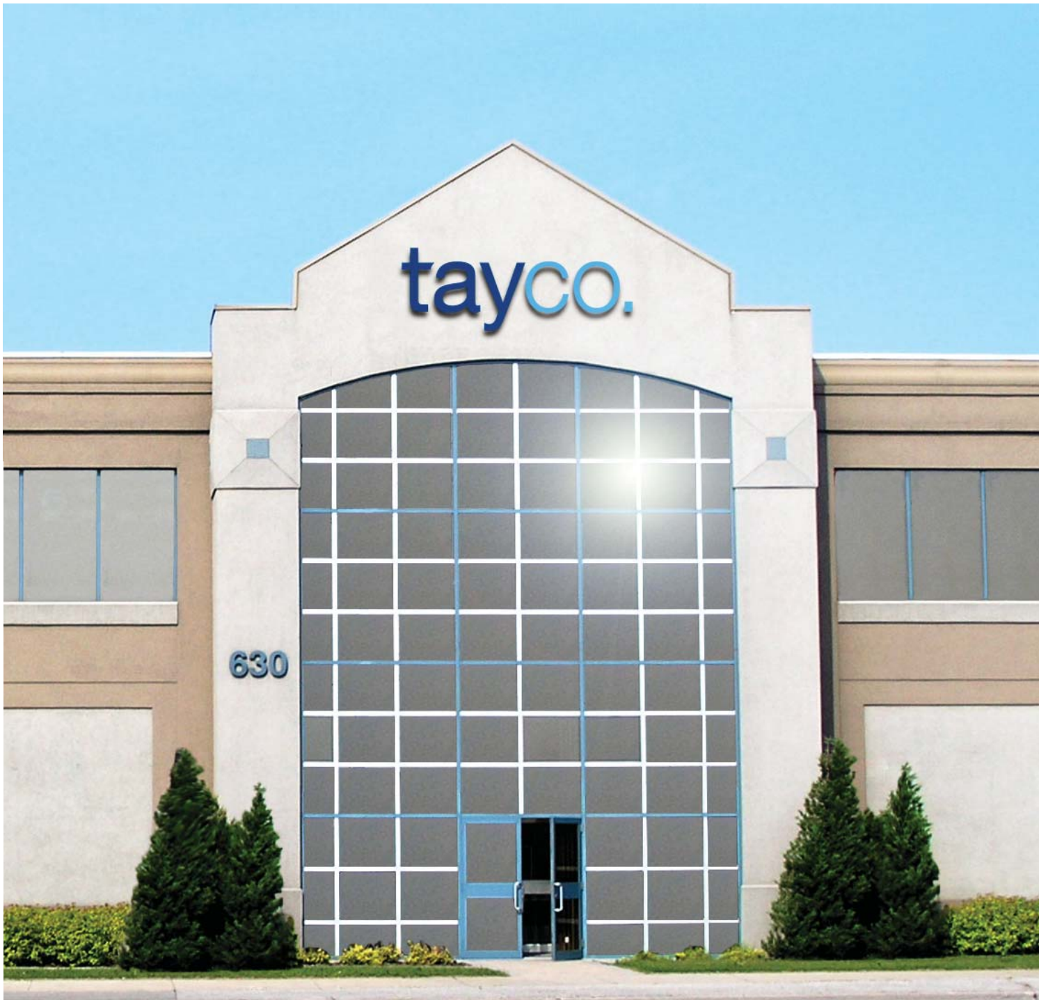
Head Office, 630 Kipling Avenue, Etobicoke
