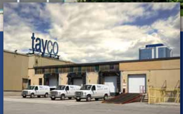
Manufacturing Facility, Norris Glen building, Toronto
